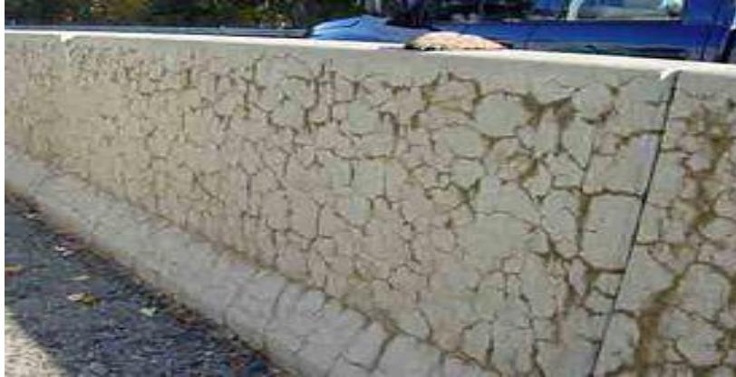
Typical effect of Alkali-Aggregate Reaction
