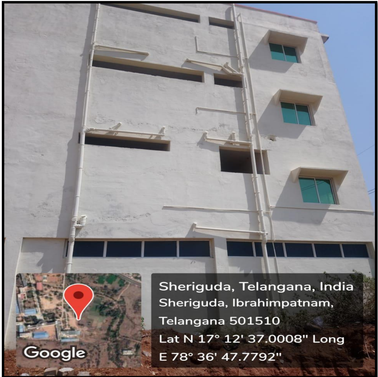
Waste water pipelines
