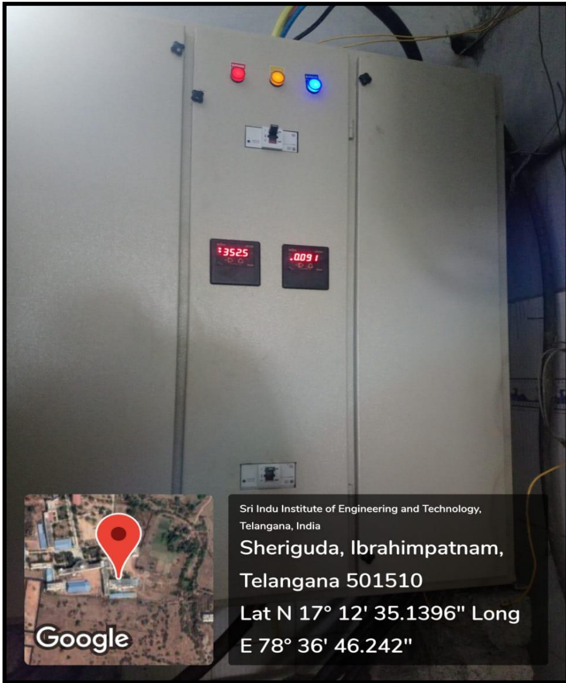
Net metering connection
